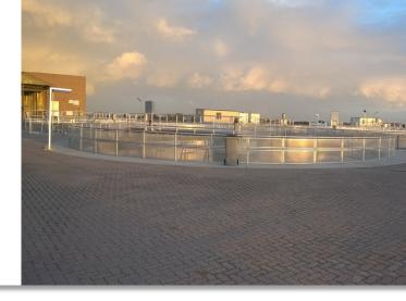
SA Water's Glenelg STP processes wastewater from the south west region of Adelaide, with a capacity of to the equivalent of 200,000 persons or up to 60MLD.
