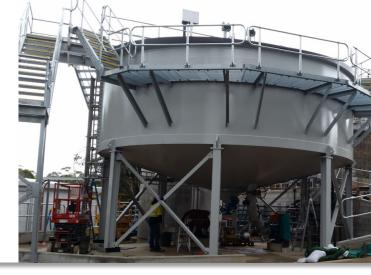
The Landers Shute WTP operated by SEQ Water was recently upgraded by Stirloch Constructions to include a new pre and post lime dosing system. A Hydroflux Epco Lime Saturator was included as part of the works.
