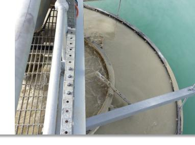
The Mt Morgan Mine WTP processes 6MLD of acid water from the sites tailings dam. The process includes for a lime dosing system and lime clarifier process.
