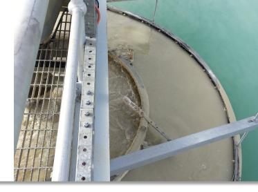
The Mt St John WWTP was upgraded in 2009 to include an advanced nutrient removal system. As part of the upgrade, Hydroflux Epco supplied 3 x 42M LogMax® secondary clarifiers and 1 x 16M VeeMax® Lime Clarifier.
