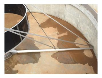
The sludge removal mechanism is fully suspended which means there is no contact with the floor. Key benefits of the HeadMax<sup>®</sup> include:
