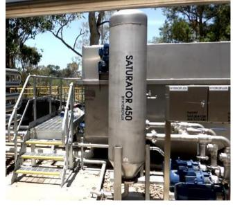
The twin dissolved air system provides a very high recycle rate and air to solids ratio
