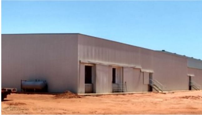
Main abattoir building under construction
