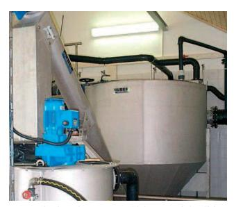
HUBER Circular Grit Trap HRSF with integrated classifying screw and subsequent HUBER Grit Washer RoSF4/t
