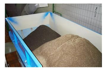
There are over 25 reference sites in Australia, and 2000 units worldwide. HUBER's grit washing technology is available in 5 sizes, with capacities from 8 through to 32 L/s of grit slurry.
