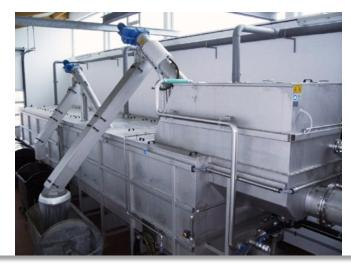
The Pemberton WWTP was recently upgraded to increase capacity and discharge quality. Part of the upgrade included a HUBER Ro5 Packaged Inlet Works.
