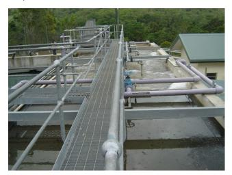
The biological system consists of a pre-anoxic tank, for nitrate removal, a single RBC unit equipped with 3 internal cascades, for BOD and ammonia oxidation, and a de-oxygenation tank for the removal of residual oxygen from the RBC unit, generating a low oxygen feed for the pre-anoxic tank.
