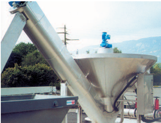
Innovative technology: COANDA Grit Washer RoSF 4 size III with frost protection for outdoor installation
