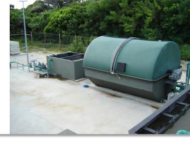
Based on successful Roadtrain<sup>®</sup> installations at Masig and Erub Is, a 100 m3/d system was installed at Mabuiag Island, located in the Torres Straits.
